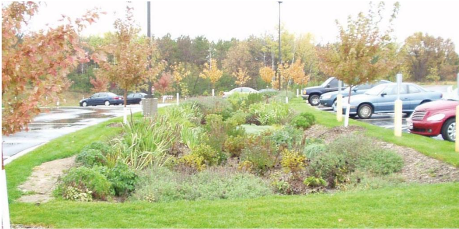
Photograph - Bioretention cells at Ithaca College capture and treat runoff from parking lots
