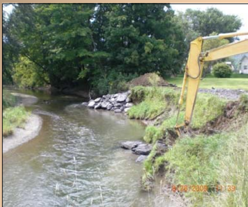
Installation of Rock Vanes, Illsley property
