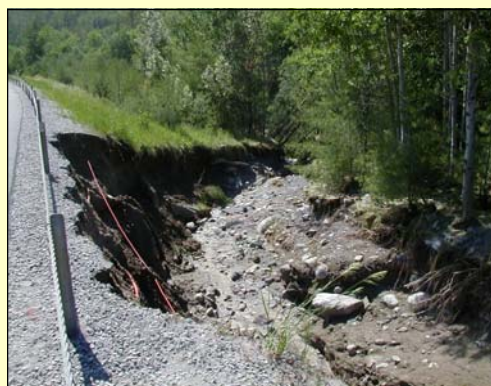
Roadside ditch erosion
