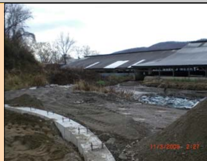
Outer ring base of slurry store constructed
