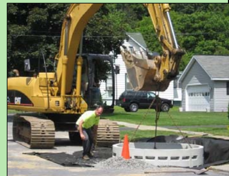
Installation of a drywell system on a Village of Lake George street in 2009
