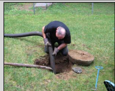
Pumping a residential septic tank
