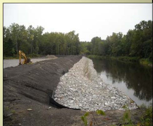
Construction of Boquet Riverbank stabilization, Willsboro Sewage Treatment Plant
