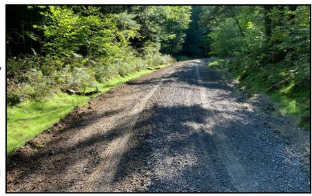
re-crowned, and graded to help with breaking up the stormwater to convey into the newly constructed swales and infiltrate the stormwater into the forest lands. Areas of open soil were stabilized with hand seeding and mulching as well as installing a series of check dams with filter sock throughout the earthen swales. The department also received a set of York Rakes from this project to maintain the road grading and project site.
